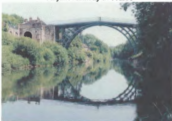
The World's first metal bridge, made from cast iron over the Severn River at Ironbridge
