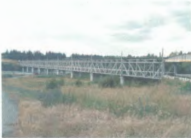
Seddon Bridge with rail crossing above and road below.
