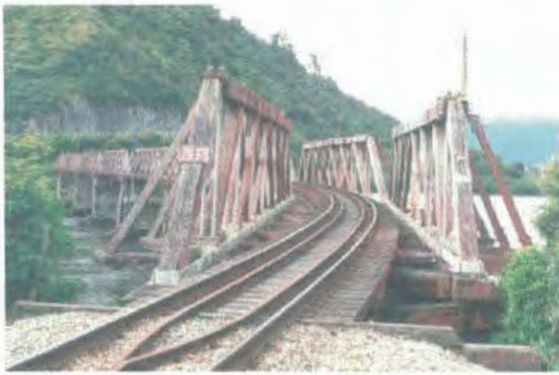
'S' shaped timber truss bridge across the Grey River.
